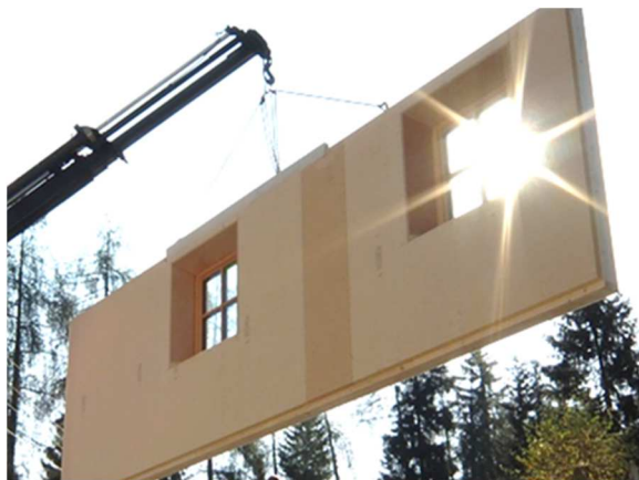
FIGURE 2-8: PREFABRICATED FAÇADE ELEMENT FOR THE THERMAL RENOVATION OF A FARMHOUSE IN TRINS [2,3]
