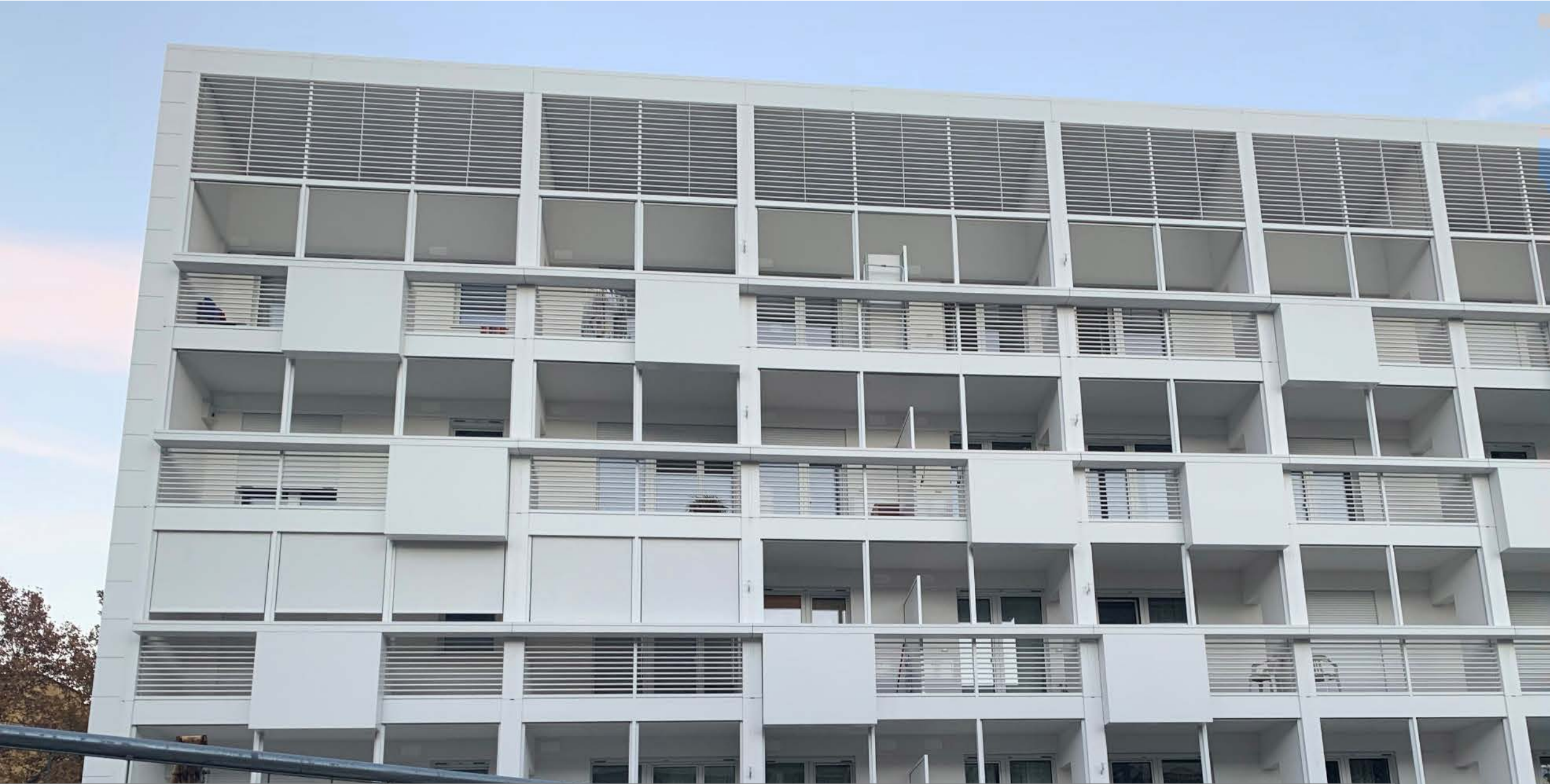
Via Similaun in advanced phase of refurbishment, IPES. Credits: Eurac Research
