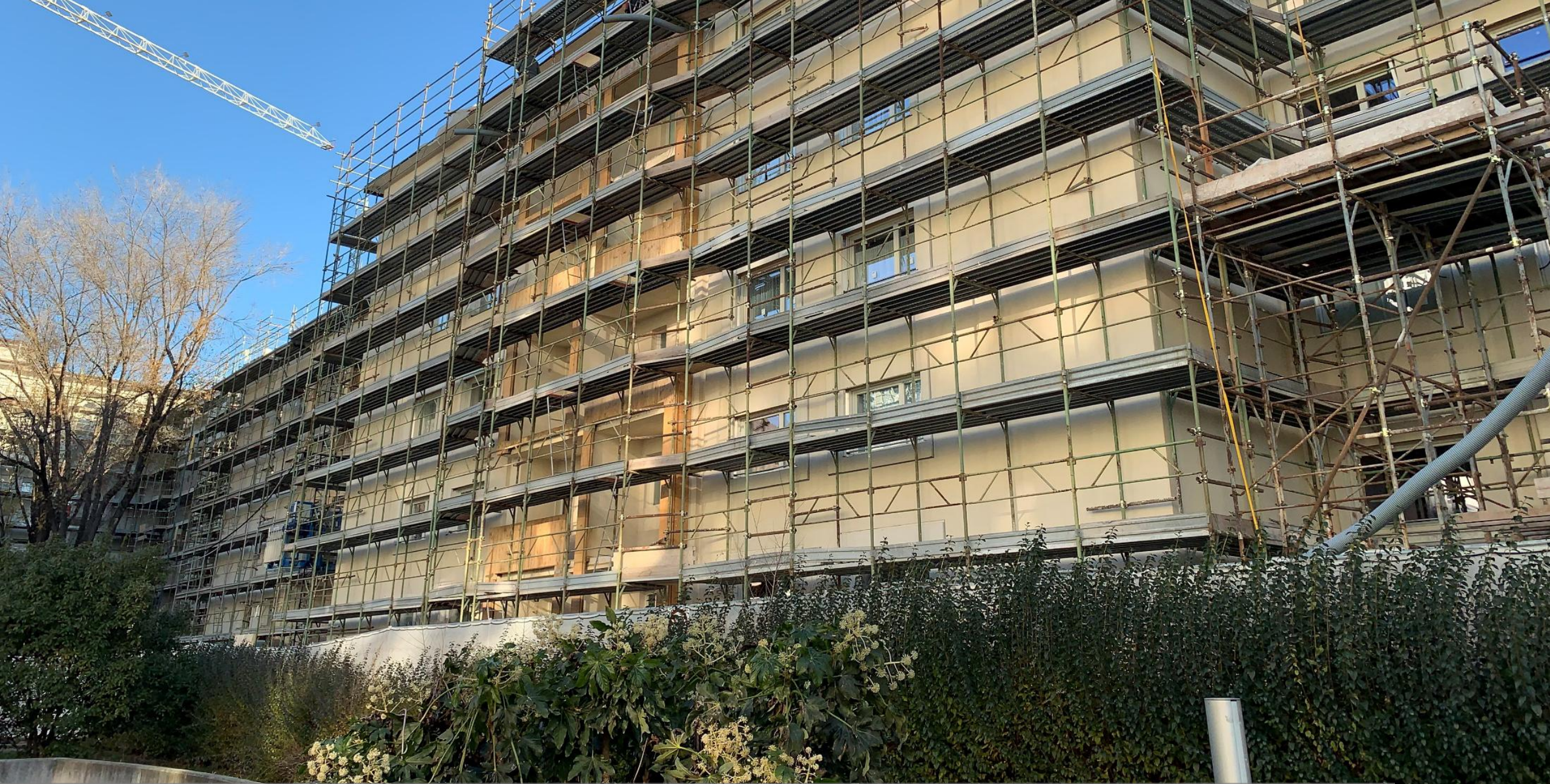
Via Palermo refurbishment works ongoing, IPES. Credits: Eurac Research
